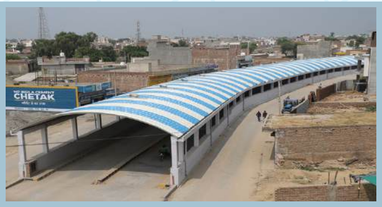
Pathway Self Supported Roof
