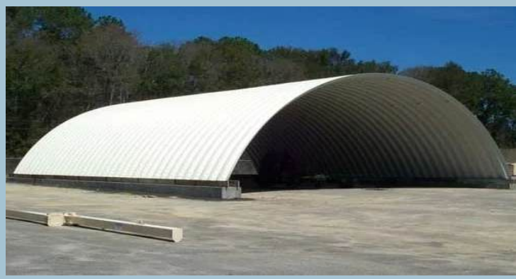
Ground to Ground Roof
