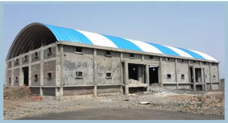
RCC Wear House
